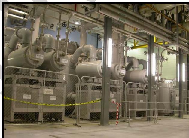
■ Figure 22 Gas Insulated Transformers
