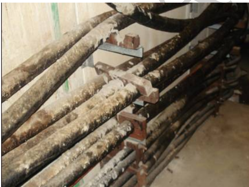
■ Figure 29 Existing Installed Paper Insulated Cables
