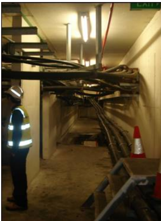
■ Figure 28 Existing Cable Congestion
